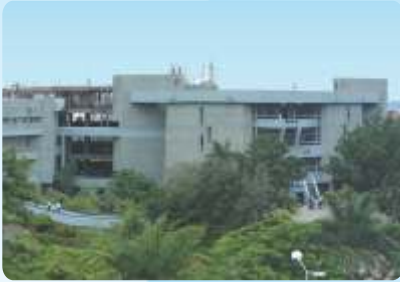
College of Engineering, Pune
